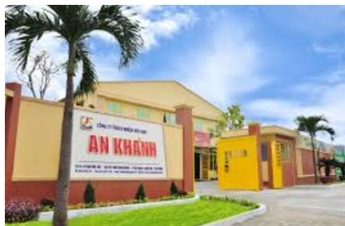
NM An Khánh An Khanh Plant
